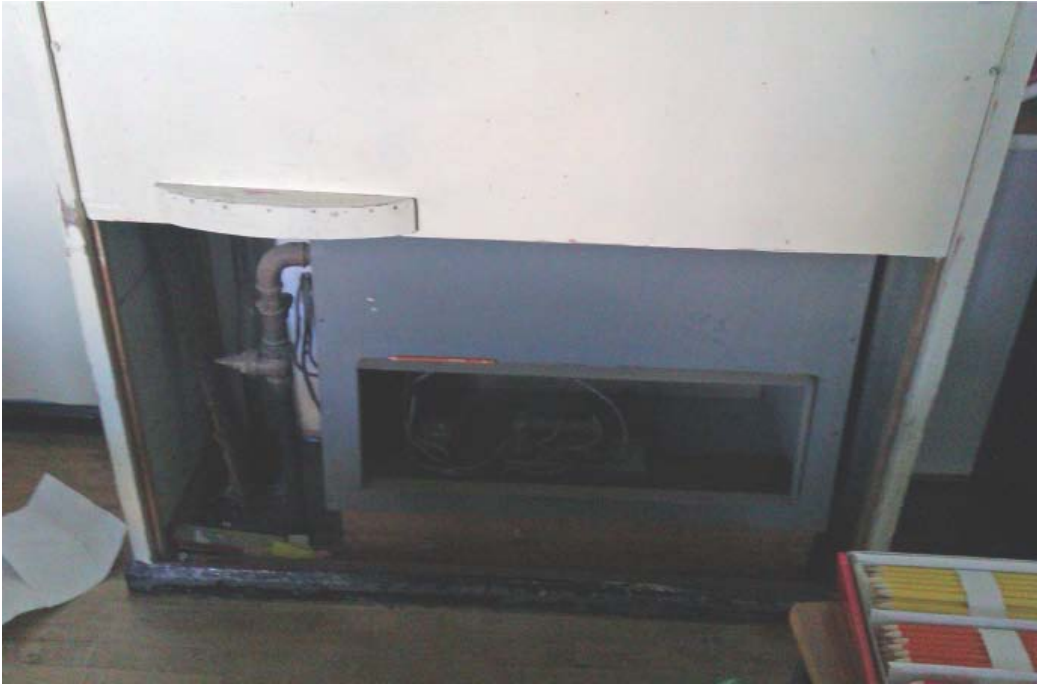
Base of free standing heater. Note front panels removed for cleaning and maintenance
