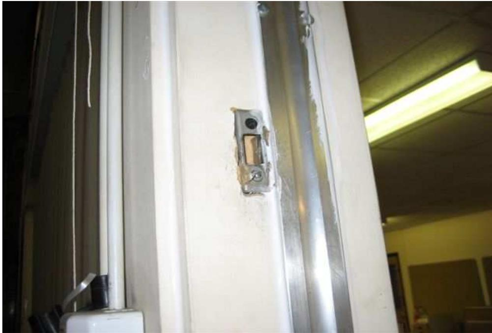
**Plate 16: After remediation. The cracks in the columns have been sealed. However the ceiling tiles are ill fitting.**
