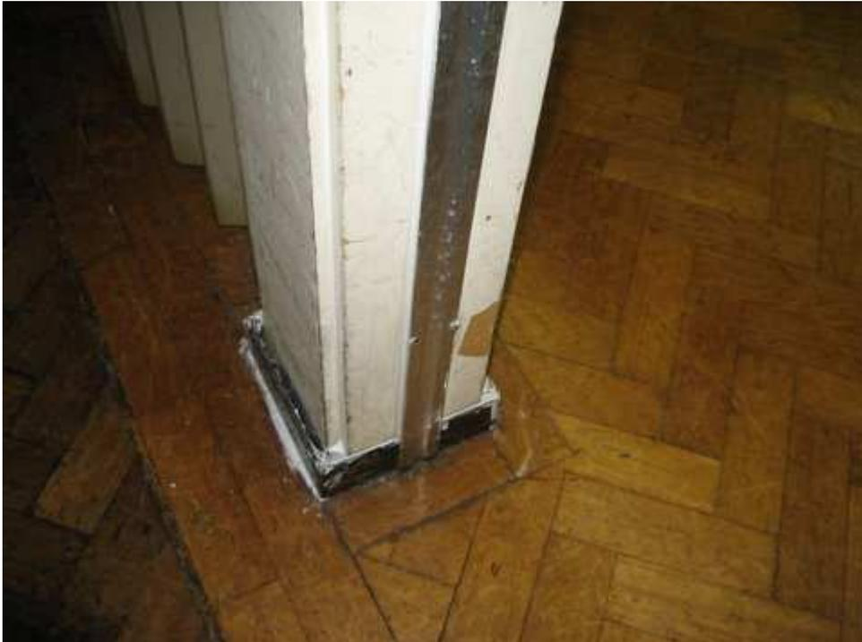
**Plate 15: After remediation. All the fittings remain in place with silicone sealant liberally applied around the edges.**
