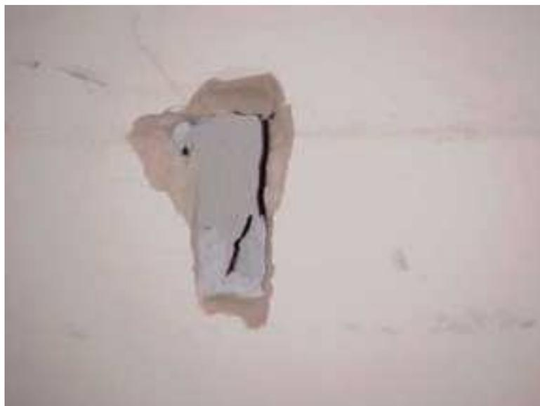
377. Having identified the problem HSE, LGE, DfES and Scape all recommend that the gaps in the skirting boards and walls should be sealed as well as the open tops of the wall voids:
