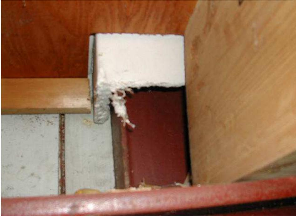
Note: It appears that the asbestos cladding has been cut when fitting the shelves. This would release large amounts of asbestos fibres. It is possible that this is moulded cladding.
