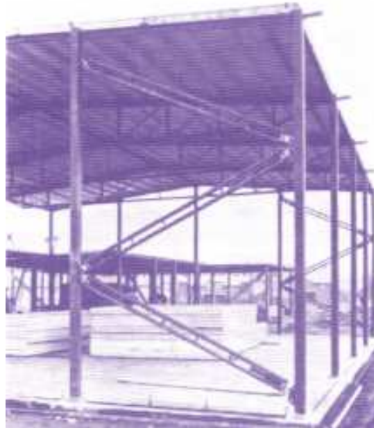
Plate 1: System Build Steel Structural Frame
